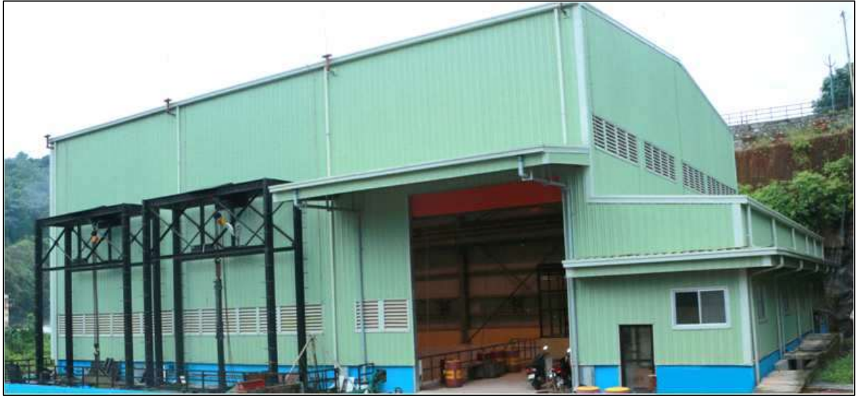
Fig 1.12: Power House – Perumthenaruvi SHEP
