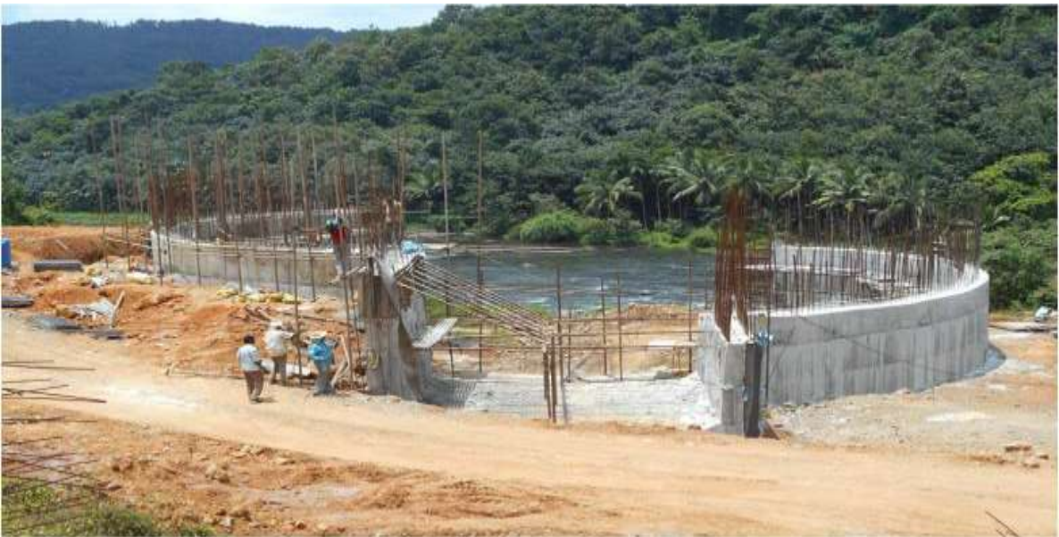
Fig 1.10: Fore bay tank during Construction
