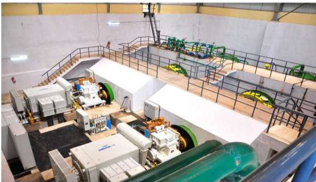
Fig 1.14: Power House during Construction stage
