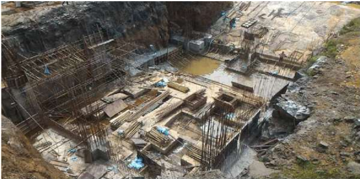
Fig 1.13: Power House during Construction stage
