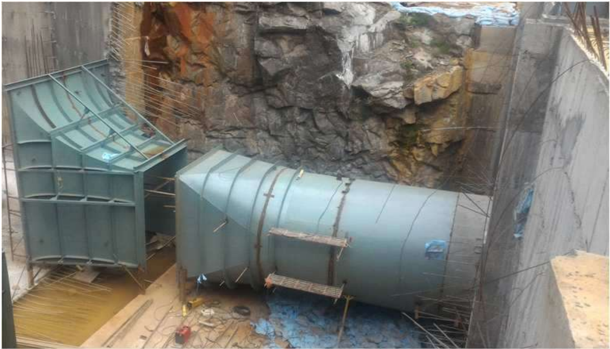
Fig 1.11: Penstock during the Construction
