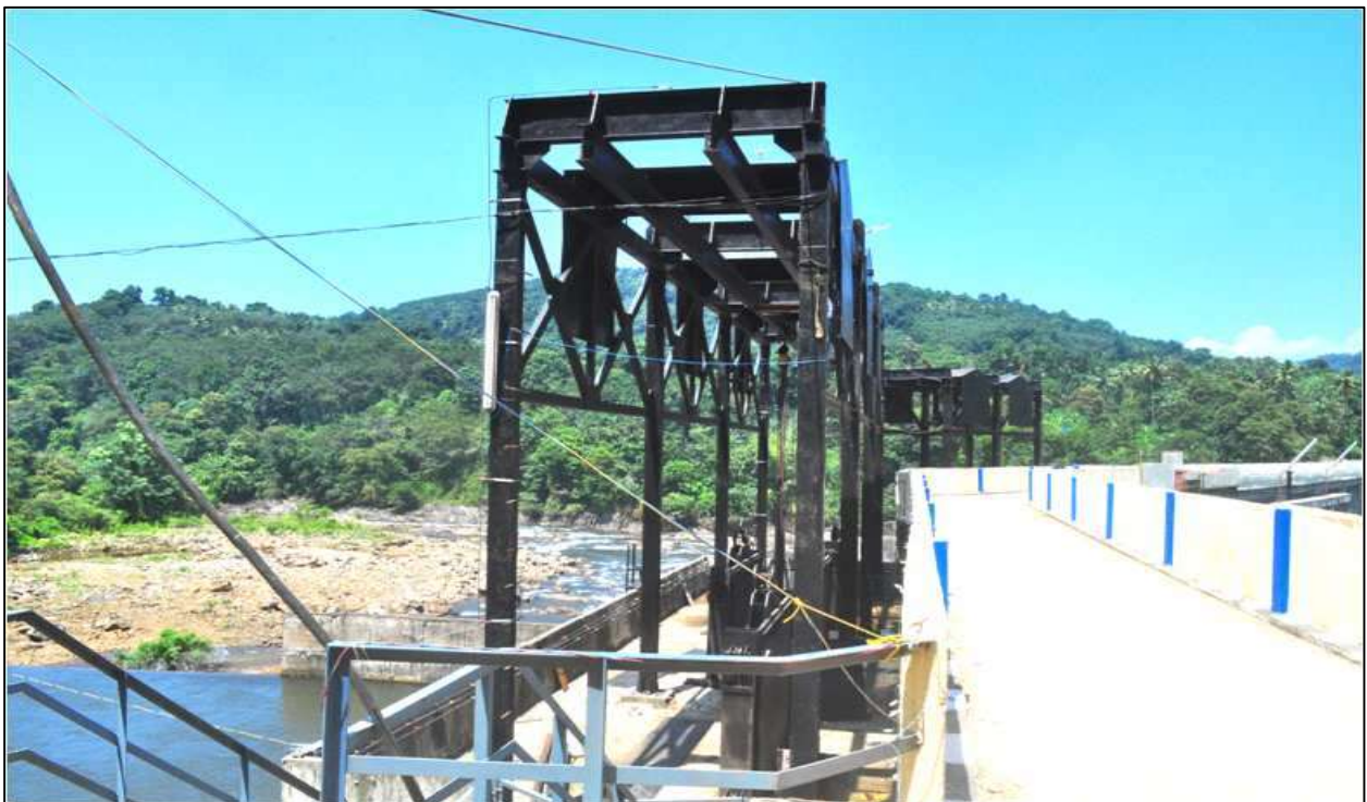
Fig 1.6: Intake and Sluice arrangements
