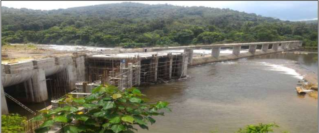
Fig 1.7 : Intake and Sluice arrangements. Photographs at Construction Stage
