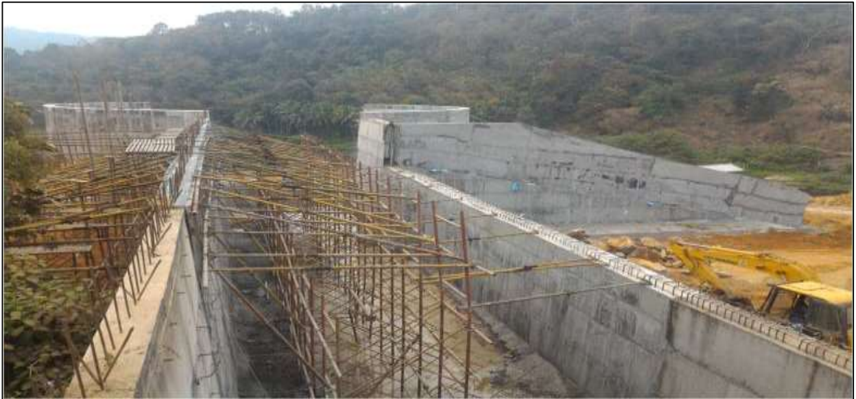
Fig 1.8 : Power Channel during Construction
